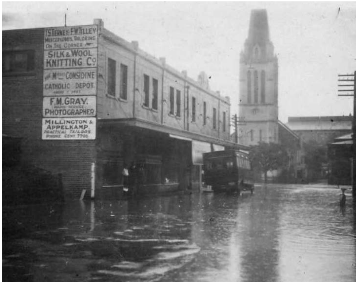
Flooding in Gawler Place South after the downpour of 6 February 1925. See also photograph of Victoria Square, p. 103. Photo courtesy of The Advertiser.
