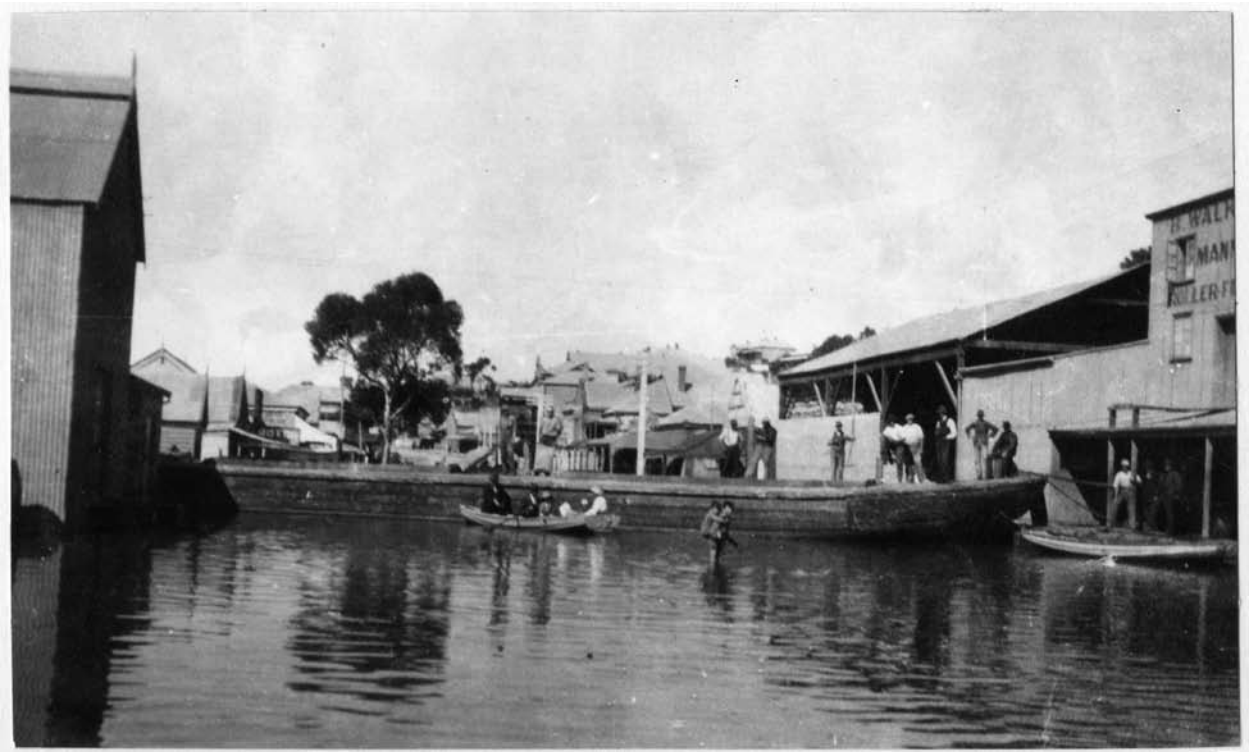
In 1917 at Mannum, a barge was floated across the main street to act as a temporary footbridge. Courtesy of the State Library of South Australia. PRG1258/2/992
