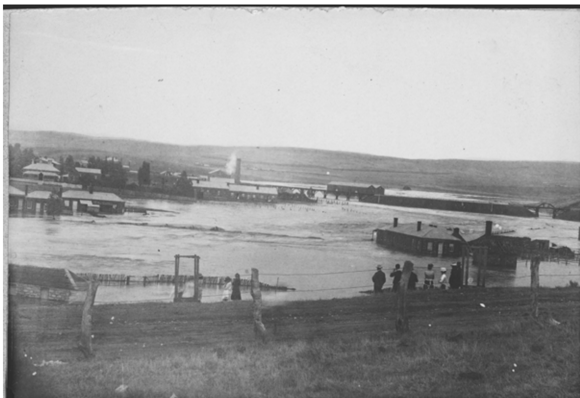
Flood at Burra, ca1899. May refer to chronology entry for 24–27 March 1899. Courtesy of the State Library of South Australia. B11558
