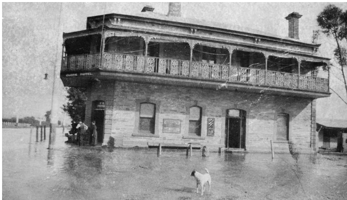
Sturt Creek floodwaters at corner of Brighton Road and Pier Street, Glenelg, ca1918. May refer to chronology entry for 19–24 July 1917. Courtesy of the State Library of South Australia. B20677
